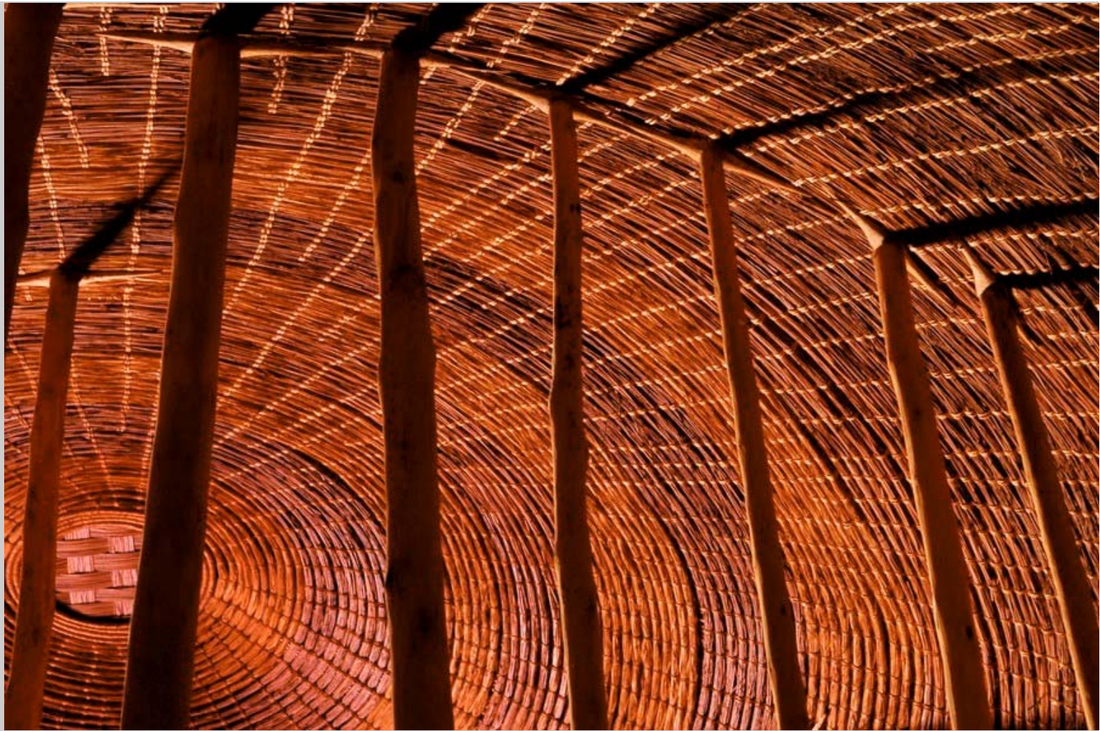
Ceiling and supports
